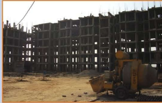
Actual Site Photograph of Avalon Residency, Ph. I, Bhiwadi
